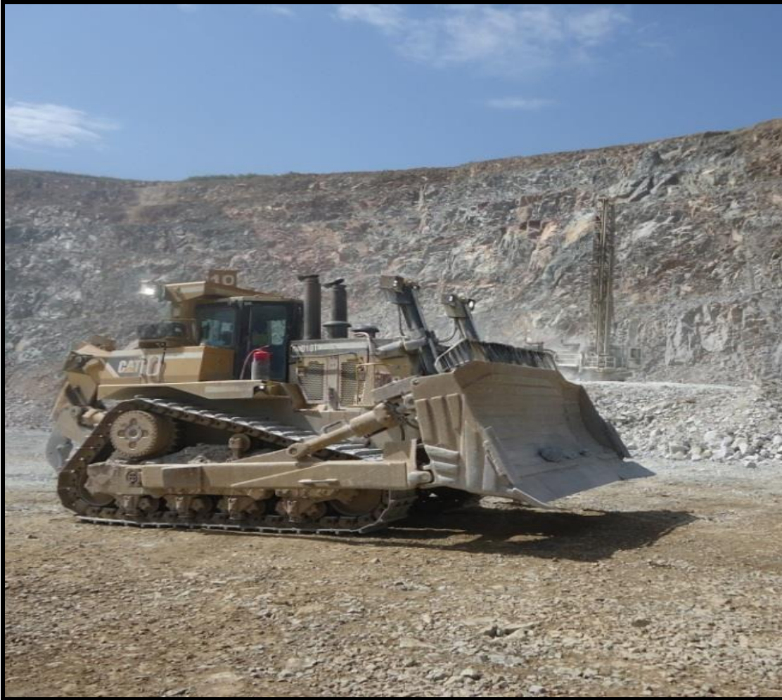
Figure 3.7: Dozer machine used for pushing materials
