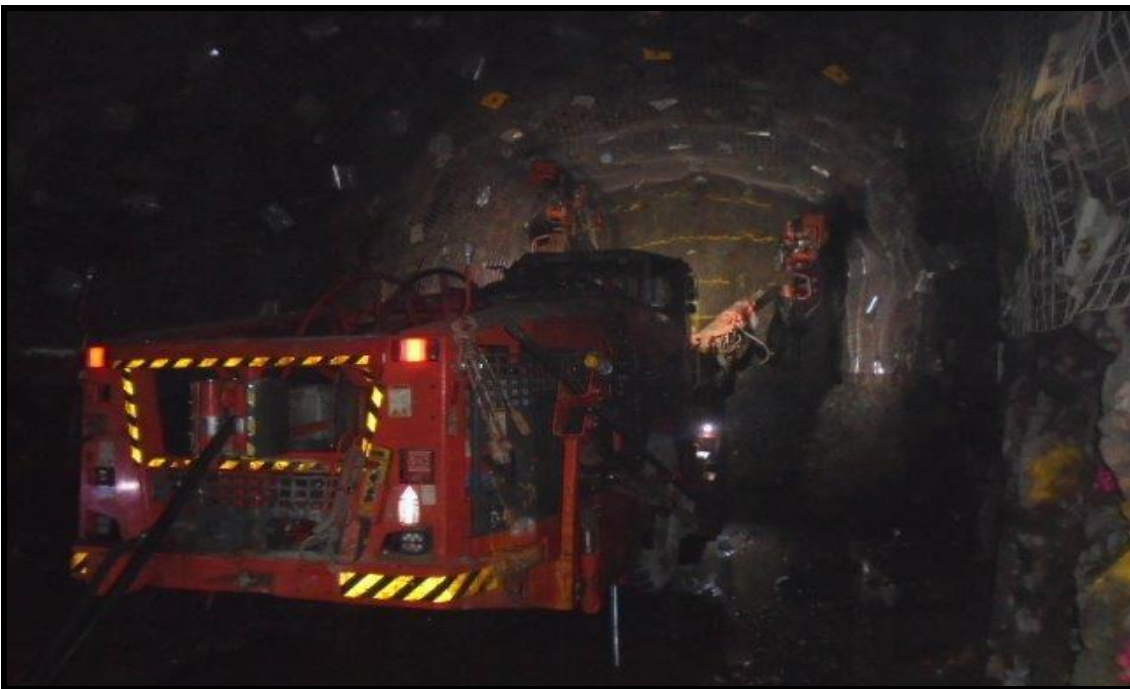
Figure 3.5: Jumbo machine used for drilling underground
